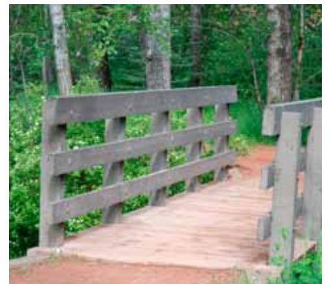
Bridge over the Big Hill Springs Creek
